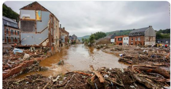
edition.cnn.com Enormous scale of destruction is revealed as water subsides after historic western Europe flooding
